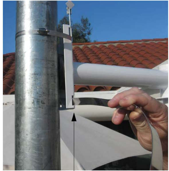
Feed strap through bracket
